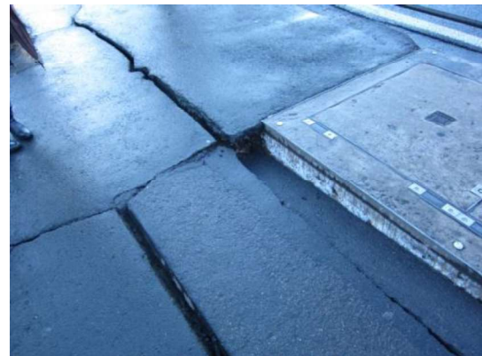
Cracked and heaved pavement
